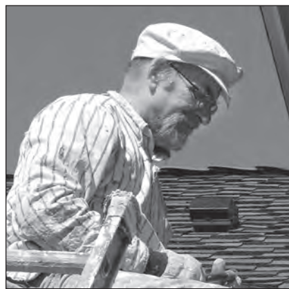
Volunteer Will Larsen working under the eaves
