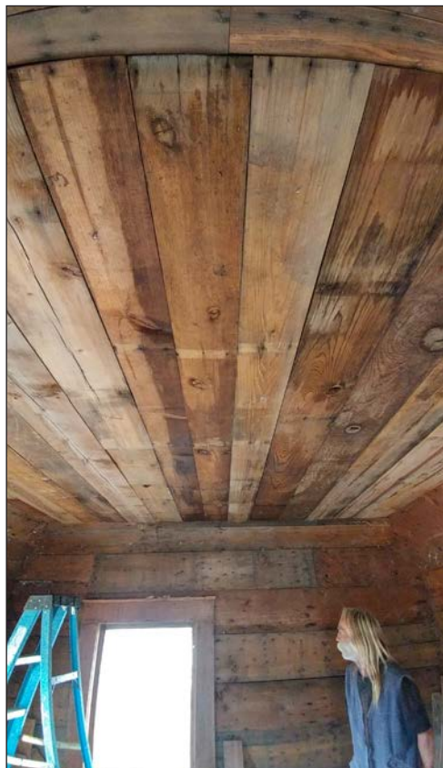
Rick Nicely works on the cabin’s interior.
