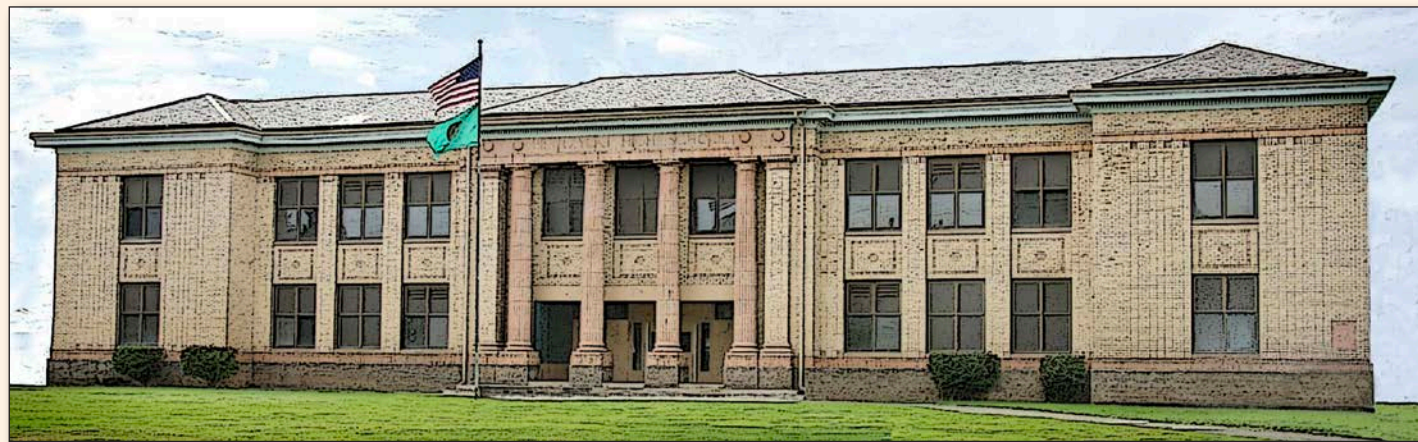
This is an artist's rendition of the Pietrzycki High School, which is currently under construction. It will be finished for the 1923-1924 school year.
